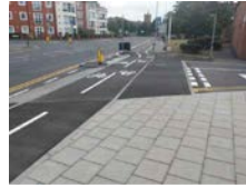
FIG - 2: EXAMPLE OF SIDE ROAD ENTRY TREATMENT - PARTIAL SET BACK CONTINUOUS FOOTWAY AND CYCLEWAY CROSSING
