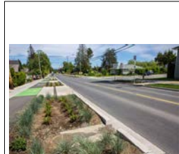
FIG 1 - EXAMPLE OF LOW-LEVEL VEGETATION ON THE HIGHWAY SOURCE: https://www.courtenay.ca/EN/main/community/downtown-revitalization/5th-street-complete-street/5th-street-rain-garden.html ACCESSED ON 18/08/22
