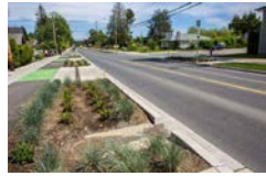
FIG - 1: EXAMPLE OF LOW-LEVEL RAINWATER GARDEN
