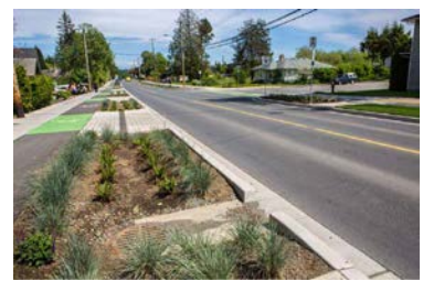
FIG - 1: EXAMPLE OF LOW-LEVEL RAINWATER GARDEN
